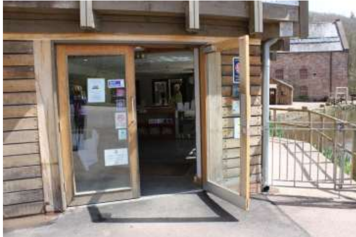
Entrance doors to the Centre
