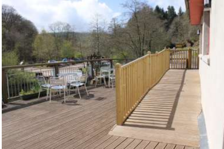
Access to the café decking is via a wooden ramp at the front of the Centre
